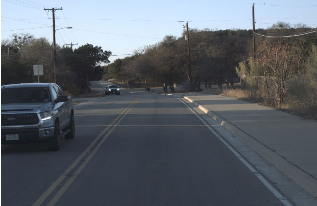
Figure 7: COMANCHE GAP RD (PCI=98.7, Good Condition)
