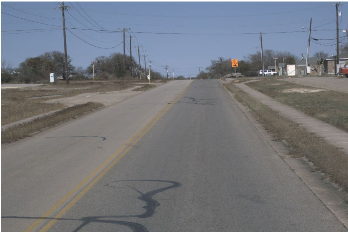
Figure 10: INDIAN TRAIL DR (PCI=76.3, Satisfactory Condition)
