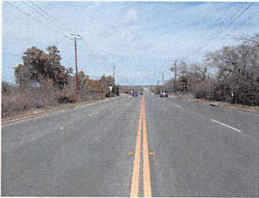
Roy Reynolds Drive North of VMB 1-inch Asphalt Overlay
