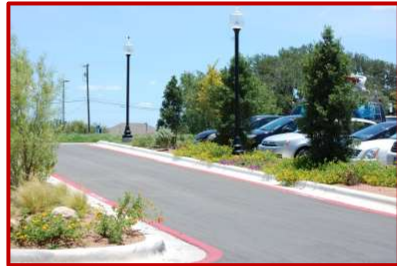
Figure 51 - Parking Lot Lighting
