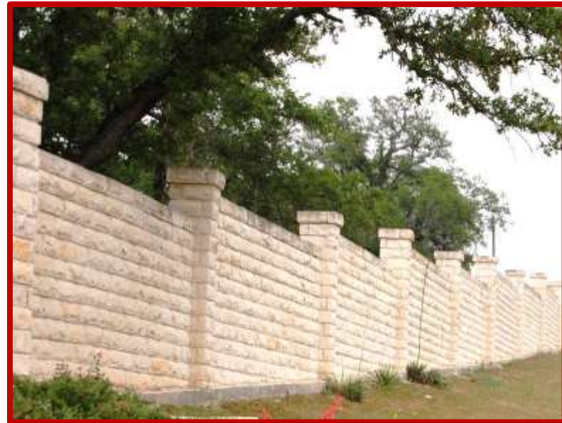
Figure 76 - Masonry Screening Wall
