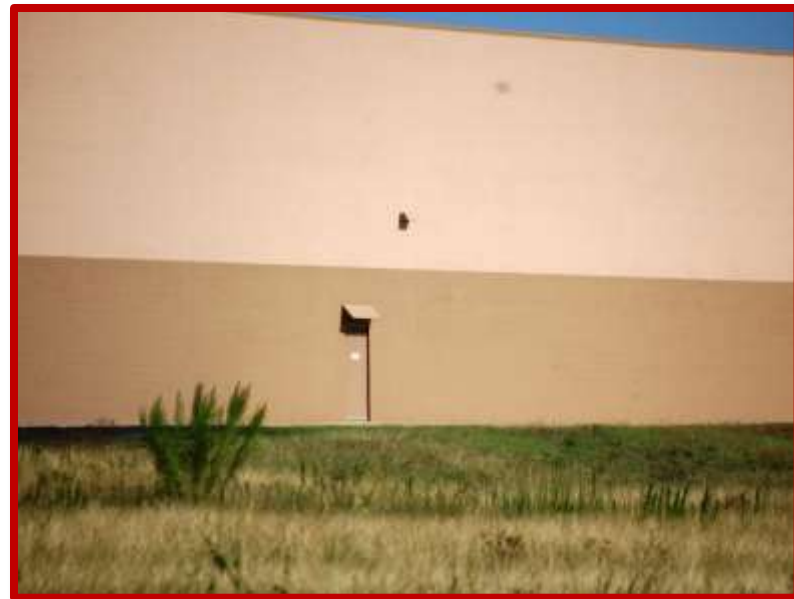
Figure 85 - Blank Walls Visible by the Public Are Prohibited
