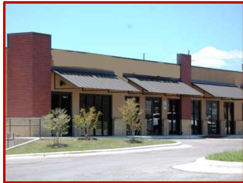
Figure 97 - Awning Extends Across Entire Walkway
