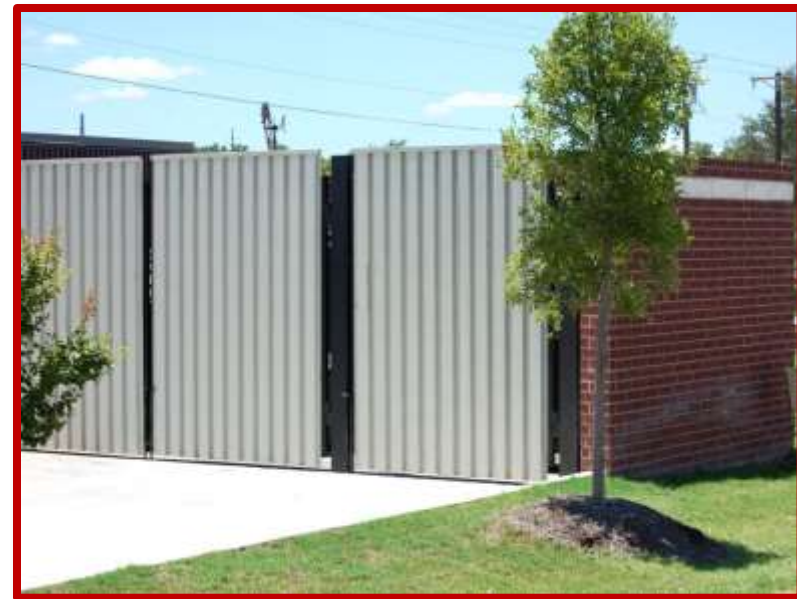
Figure 55 - Enclosed Dumpster with Appropriate Gate
